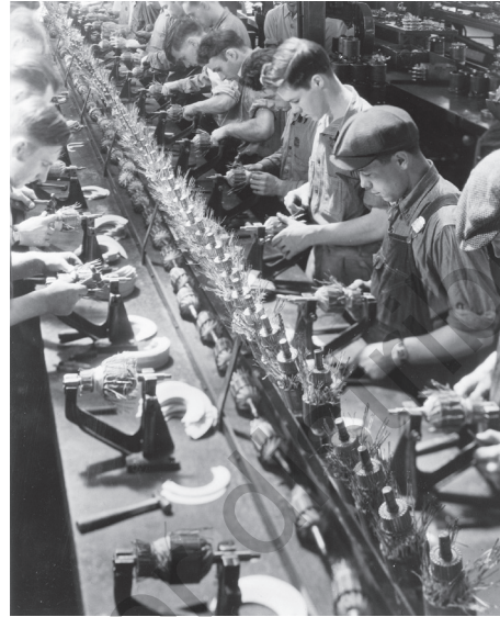
The production line is a classic example of technological control.
