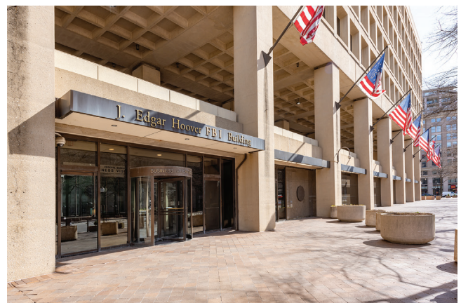
The J. Edgar Hoover building, headquarters of the FBI, in Washington, D.C. Up until 2020, annual UCR was compiled by the FBI after local, county, and state criminal justice agencies sent in their annual crime data.
